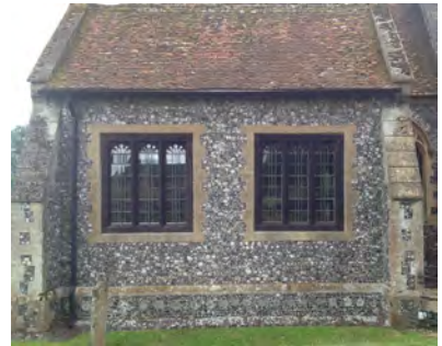
The Englefield Chapel with its modern flint walls and original-style square-headed windows
