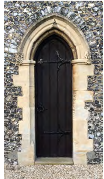
The narrow west door from the outside. It is now covered on the inside
